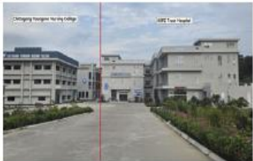
KEPZ Trust Hospital
