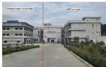
KEPZ Trust Hospital
