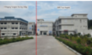
KEPZ Trust Hospital
